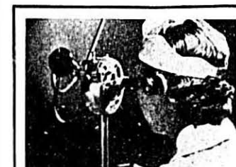
This scientific instrument is the Zeiss refractometer. It is used in all Armour egg plants to determine the solids content of every can of Cloverbloom Frozen Eggs.
